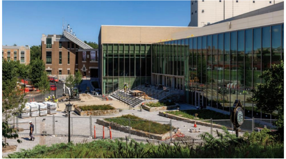
Pictured: Work on Hoag Pavillion nearing completion
