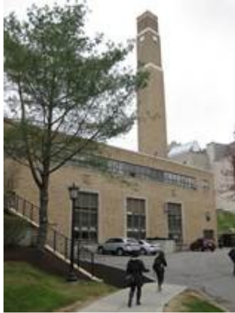
Figure 1: BC's Central Heating Plant houses one boiler field-erected in 1967 rated to produce 35,000 pounds of steam per hour and two boilers from 1979 rated to produce 50,000 pounds of steam per hour.
