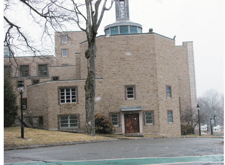
View of the Chapel
