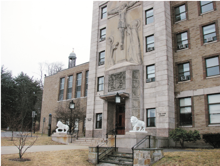
View of the Main Entrance
