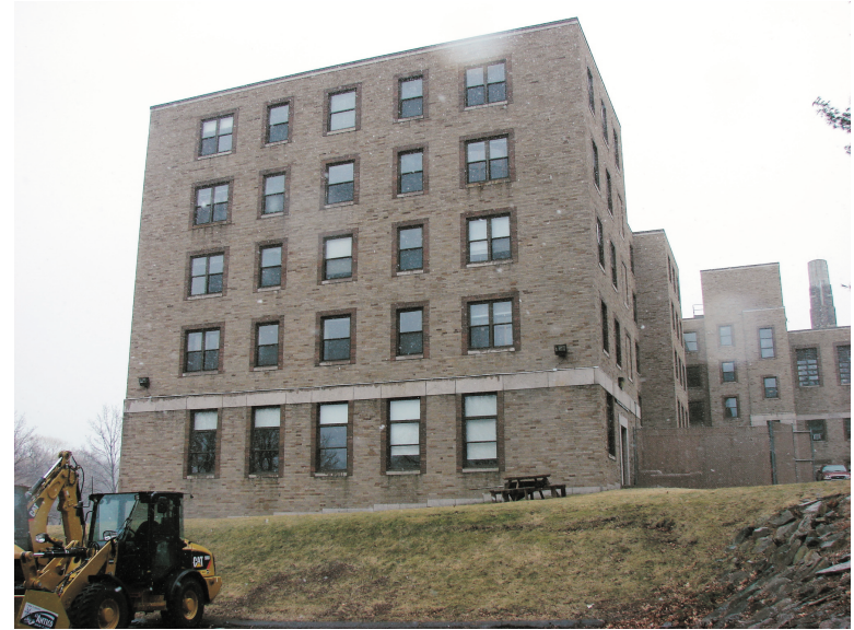
View of the North Wing
