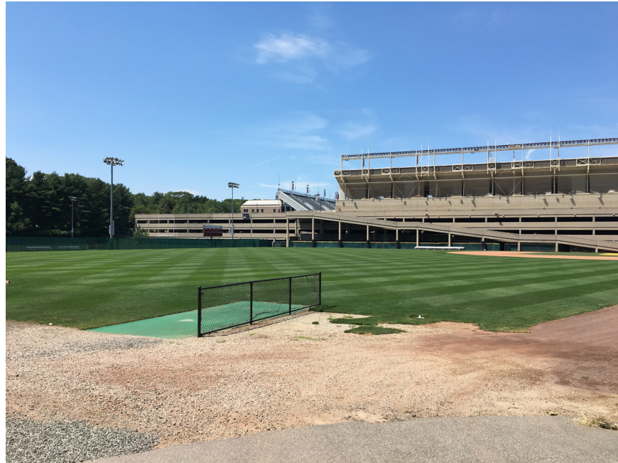
View of Beacon Street Parking Garage, Practice Field and Shea Field, east elevation from Pine Tree Preserve, facing SW
