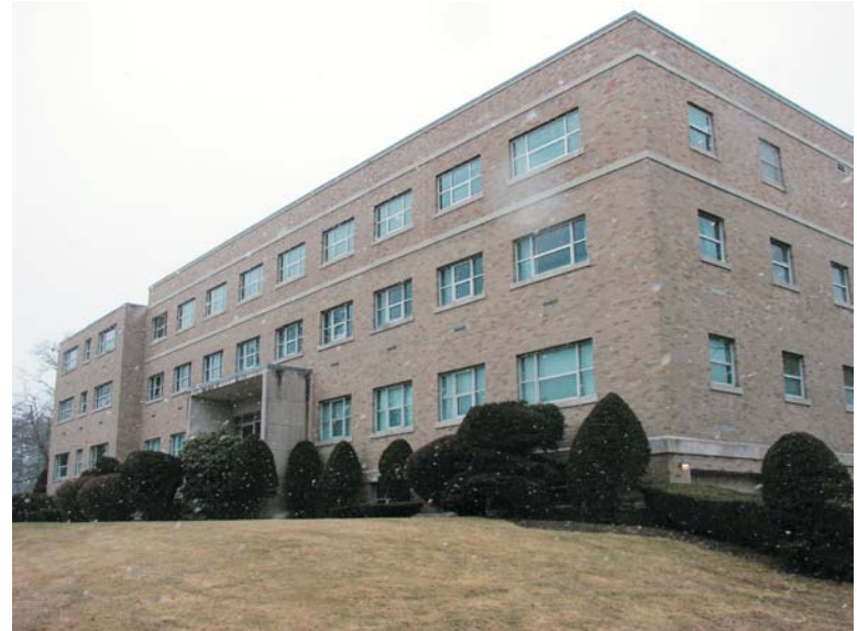
View looking Southwest of the North Wing
