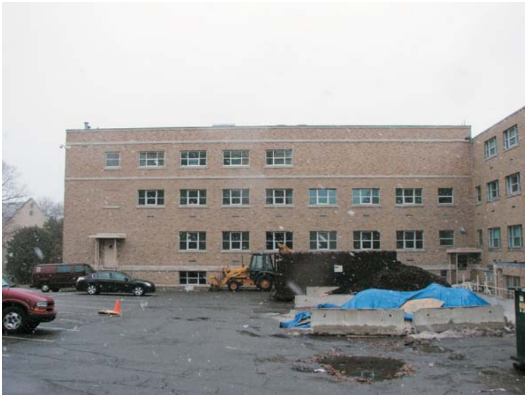
View looking East of the North Wing
