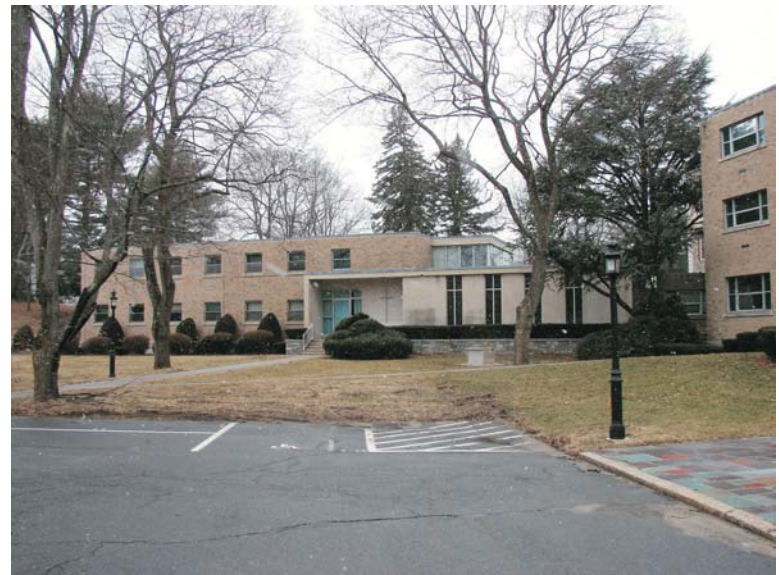
View looking West of the Building to be Demolished
